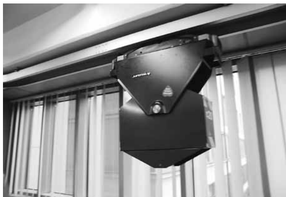
Obr. 2. Systém na transport kníh – Unicar-Telelift
